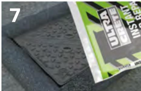
Apply UltraCrete Instant Road Repair® cold lay asphalt concrete using a 50% surcharge, compact to the required depth (typically 45mm layers, compacted to 30mm)
