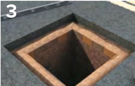
Old bedding mortar, loose bricks and debris are removed
