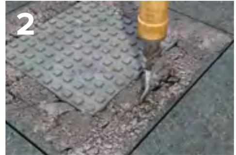
The picture frame is saw cut and excavated and the existing cover and frame removed
