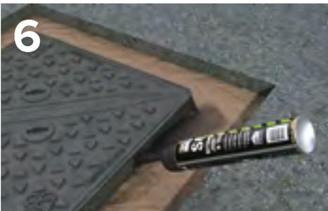
Spray all vertical edges and substrate (including manhole frame) with UltraCrete SCJ seal and tack coat spray
