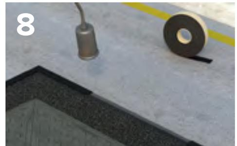
Once the Instant Road Repair is compacted level with the existing surface, apply UltraCrete Instaband ECO skid resistant overbanding tape
